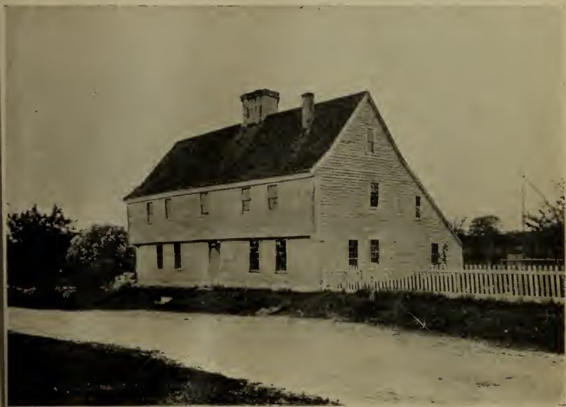
BENNETT-BOARDMAN HOUSE, OAKLANDVALE
